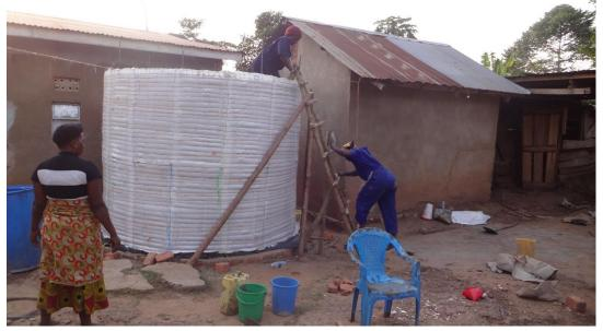
**Day six: 10<sup>th</sup> February 2019;** This marked the last activity on tank construction with plastering of tank top and application of rough-cast on tank exterior.
