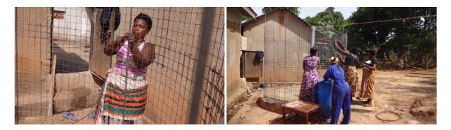
**Day four: 8<sup>th</sup> February 2019;** On the fourth day participants were taken through the second lining of the interior of the frame with a similar mixture as the first lining. They also carried out third lining of the interior which was a mixture of ordinary cement and water proof cement. This is the final lining of the interior.
